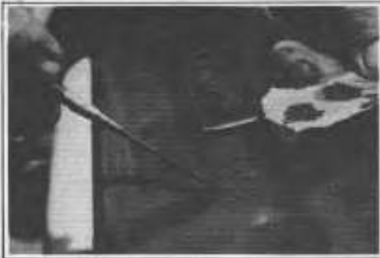
Figure 2-76. Filling Hole or Scratch
