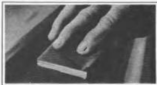
Figure 2-79. Sanding Patch
