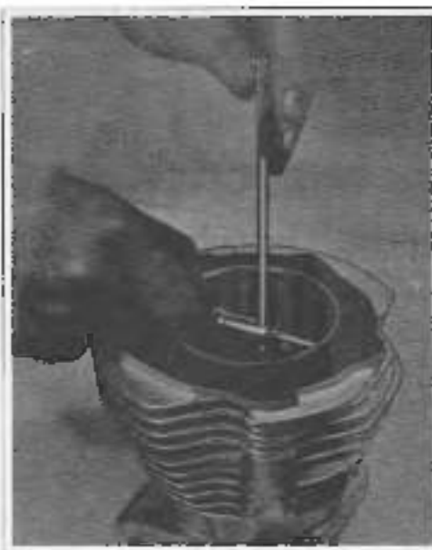
Figure 3-11. Measuring Cylinder Bore
