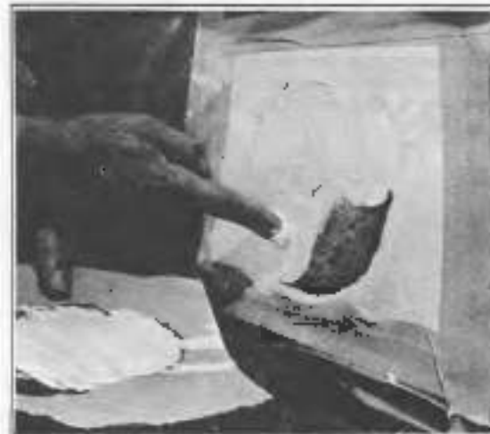
Figure 2-87. Working Gel Coat Into Patch
