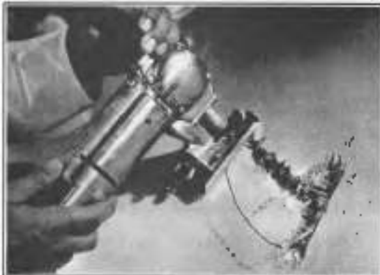
Figure 2-80. Sawing Out Damaged Area
