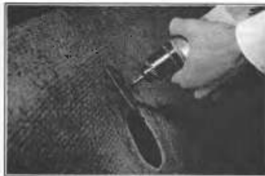
Figure 2-81. Rough Sanding Inside Surface
