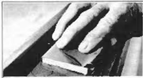
Figure 2J-6. Sanding Patch
