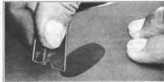
Figure 2J-5. Spreading Coat Evenly
