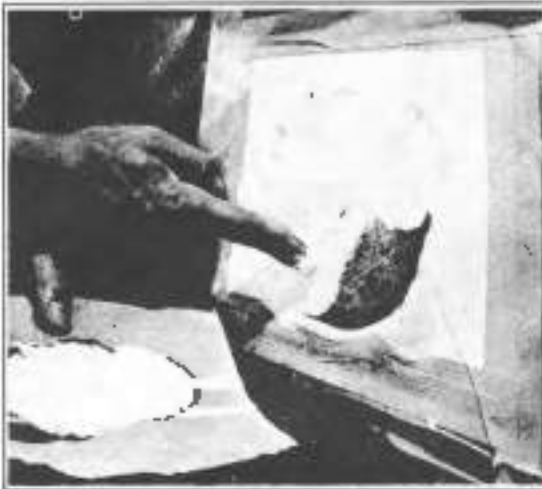
Figure 2J-14. Working Gel Coat into Patch
