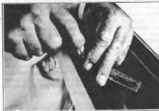
Figure 2J-4. Trimming Patch
