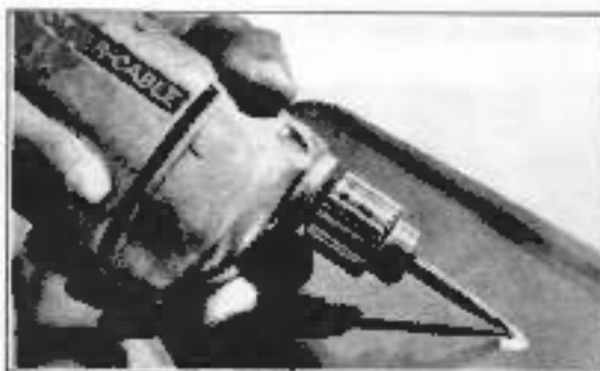
Figure 2J-1. Roughing Damaged Area
