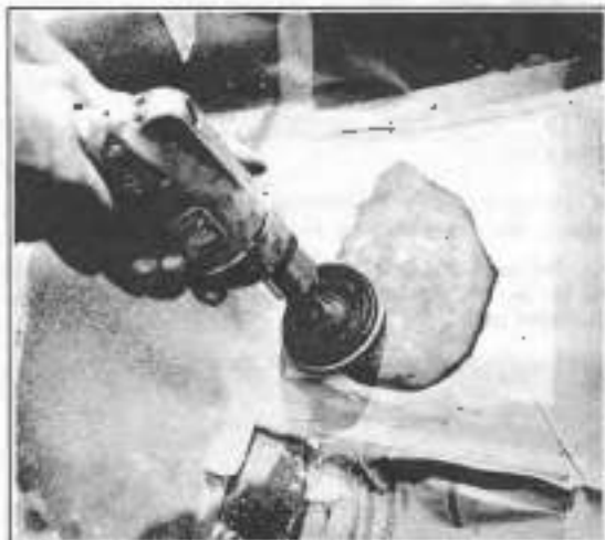
Figure 2J-13. Bleeding Patch with Sander
